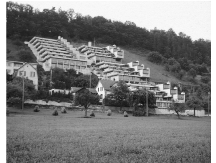
Housing project in Umiken, Switzerland by Metron (1963-71) with 30 units of hillside housing organized around diagonal elevators.
