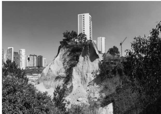
Santa Fe, Mexico City, Landslide Zone (Photo Eduardo Miranda), 2015
